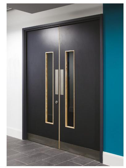
Vision panels allow users of the building to view what is on the other side of the door and are an important safety feature, vital in preventing injury resulting from collision with opening doors.
