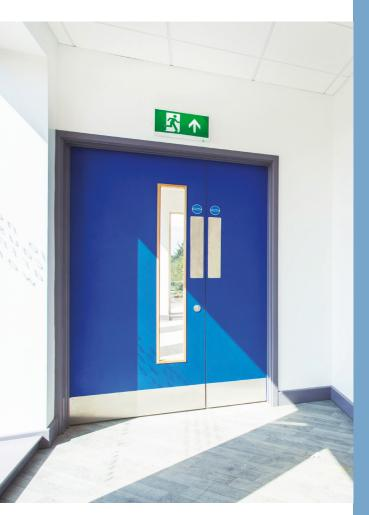
All acoustically attenuated doors require a drop seal and will also be fitted to smoke controlled doors allowing an 8mm gap below your fire door which will be sealed when door is in
