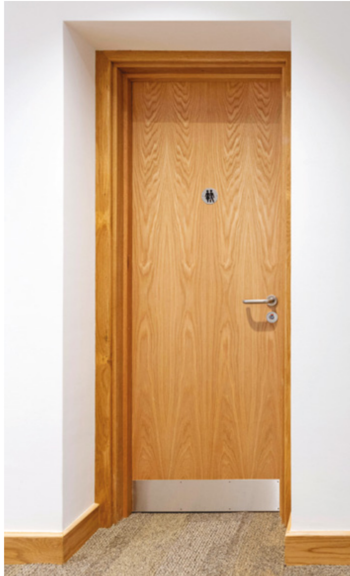
This toilet door features an American White Oak wood veneer. It also features AhmGuard integral finger protection.
