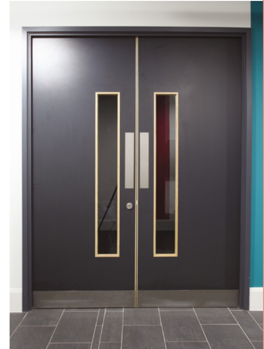
Vision panels allow students to view what is on the other side of the door and are an important safety feature, vital in preventing injury resulting from collision with opening doors.
