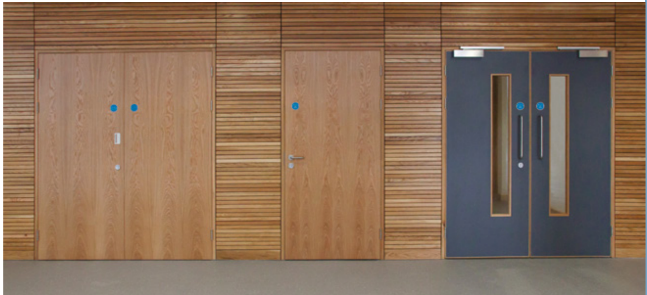
A combination of Formica Storm Grey laminate and American white oak veneered doors. Storm Grey laminate is complemented with exposed oak lippings, frames, architraves and glazing bead for circulation doors. Whilst contrasting crown cut, American white oak service and store room doors act as a way finding feature for students and teachers.
